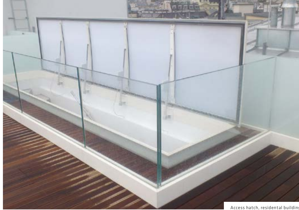
Access hatch, residential building
